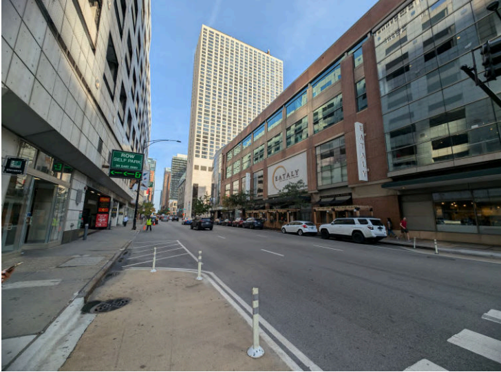
Chicago Parking Garage
